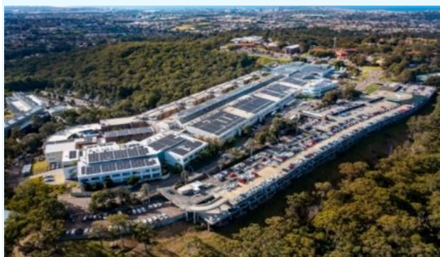
©Hunter New England Local Health District, John Hunter Hospital rooftop solar panels
