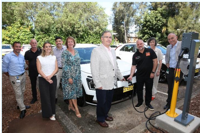
©Northern Sydney Local Health District, NSLHD Chief Executive, Board members and staff showcasing EV charging stations at Macquarie Hospital
